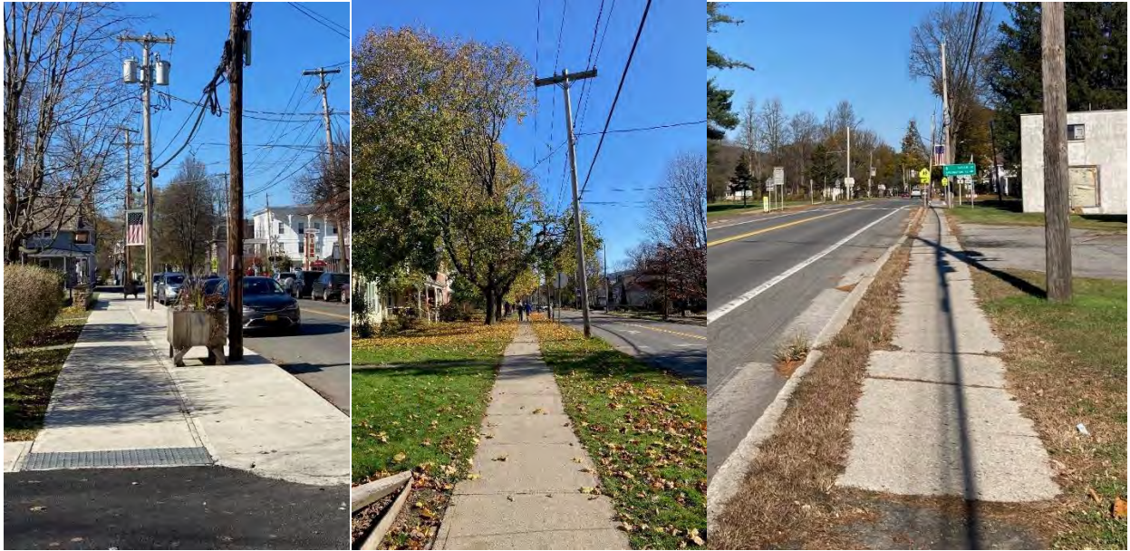
Types and condition of concrete sidewalks within the Village
