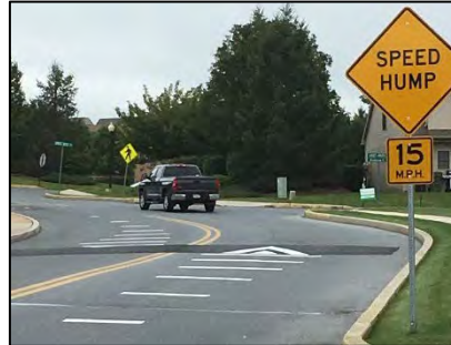
(Source: PennDOT Local Technical Assistance Program)
