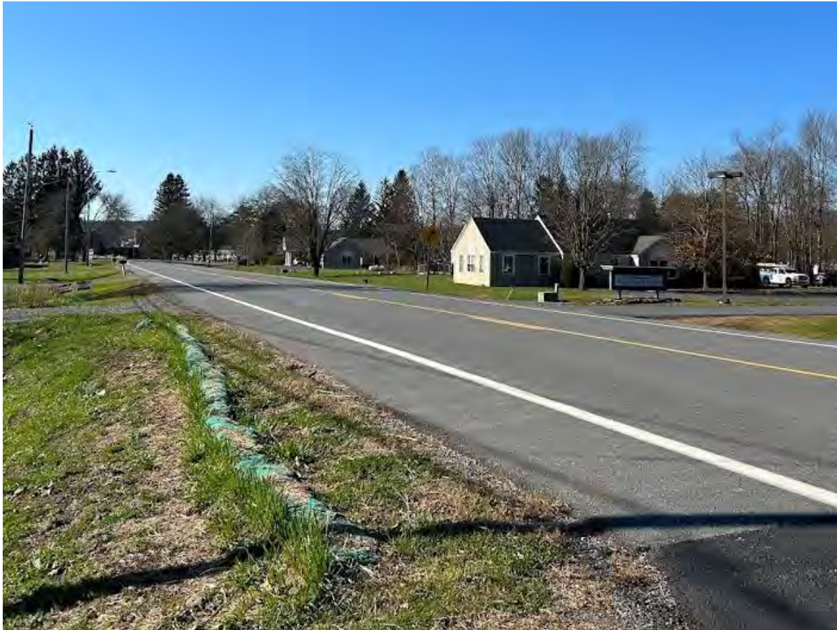
Existing Conditions on Route 313/Gilbert Street
