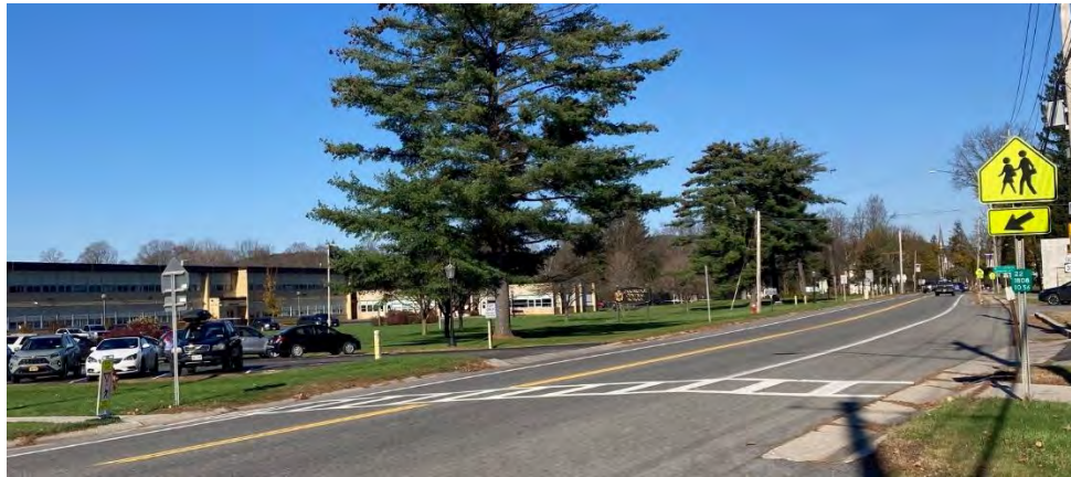
Crosswalk at Mountain View Drive without curb ramps
